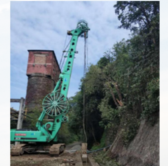
Risk control on construction site
