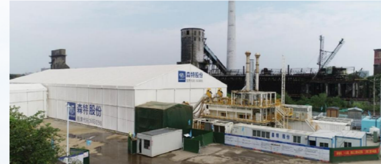
Thermal desorption disposal construction site
