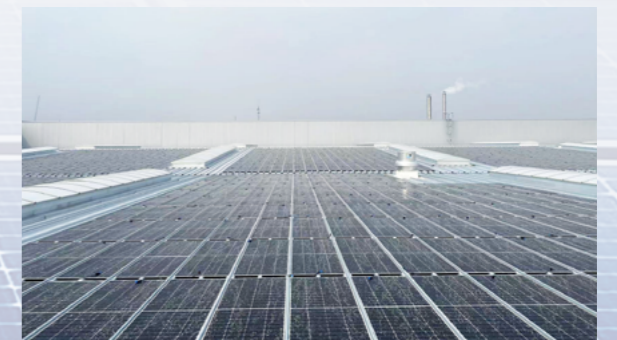
Xiaomi automobile factory project 16.2MW
